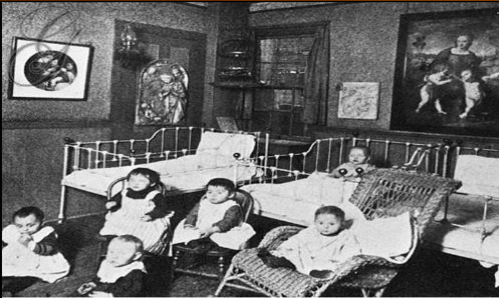
0087582 HULL HOUSE: NURSERY.
